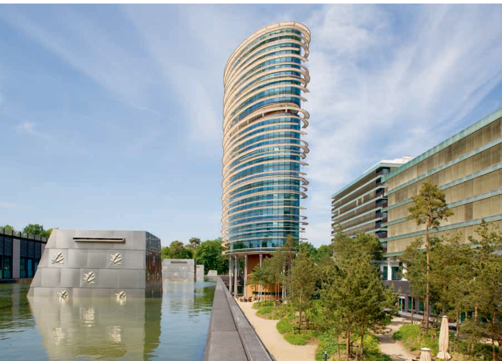
EPDM waterdak Walterbos-complex, Apeldoorn.
